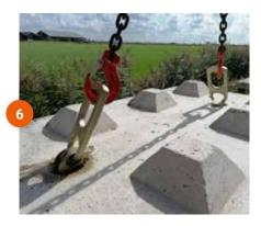
Attach the hooks to the anchors and the block is ready to be lifted
