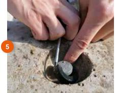
Remove the rubber from the anchor, only the top is now visible
