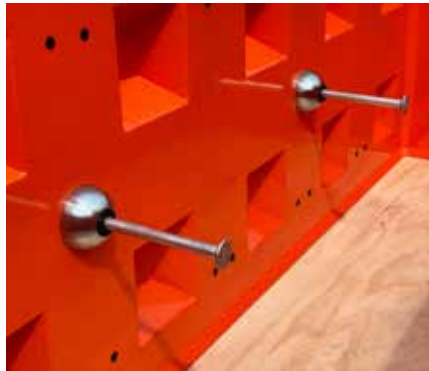
2 Place the rubber around the anchor, place the anchor in the magnet.
