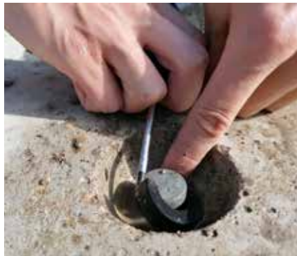
5 Remove the rubber from the anchor, only the top is now visible.
