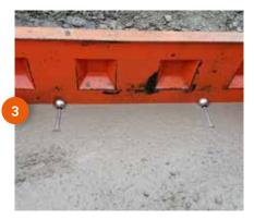
The anchor is cast in its entirety, be careful when vibrating the concrete
